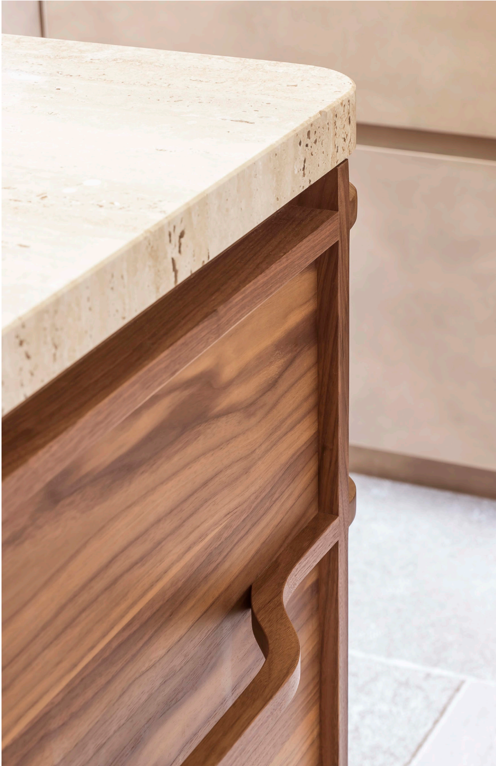
Caprini & Pellerin used solid wood so that they could carve out the handles and towel holders, creating intricate details and rounded angles in the cabinetry.
